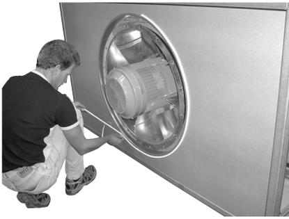
Figure 3. Fitting the sealing strip
