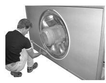
Figure 3. Fitting the sealing strip
